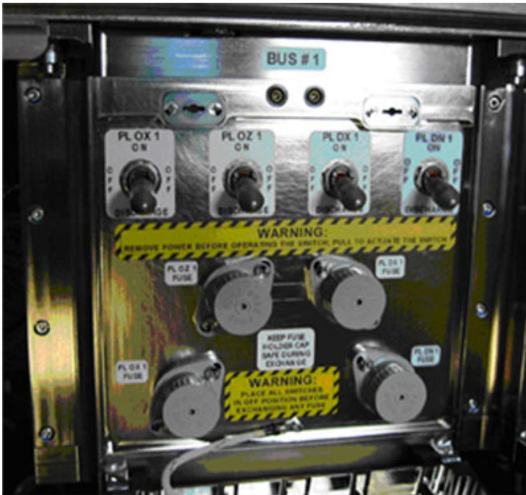
Figure 2. PPSB Bus #1 Switches (Cover Opened)
