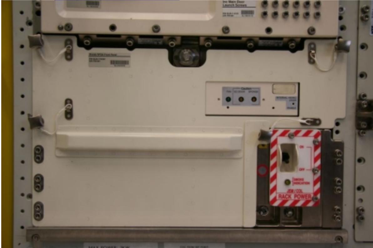
Figure 2. RPDA Panel installed
