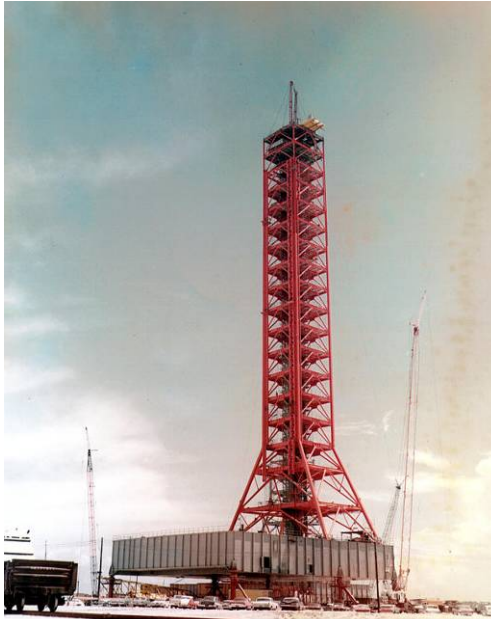
Photo 6.45. LUT and mobile launcher construction, August 1964. (Source: NASA Kennedy Space Center, KSC-64C-3077)
