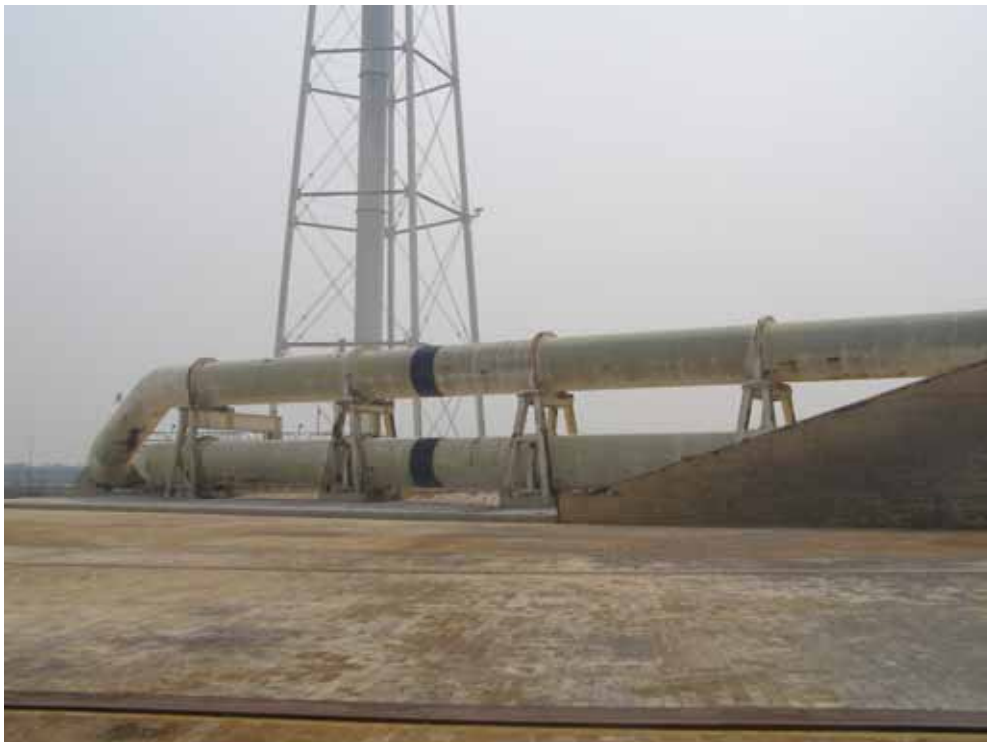
Photo 6. Launch Pad 39B, water suppression system, facing east. (Source: Archaeological Consultants, Inc., 2007)
