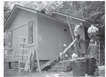
Janet's Song nearing completion
