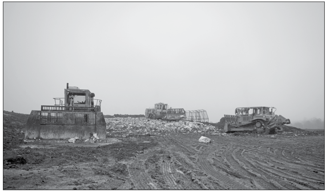
The Orange County Landfill has been open on Eubanks Road since 1972. Orange County and town officials confirmed their intent to close the landfill in 2013 at a meeting last week. PHOTO BY DUNCAN HOGE
