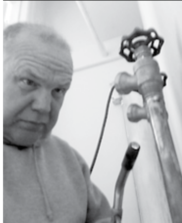
Tim Peck solders a boiler drain
