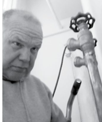
Tim Peck solders a boiler drain
