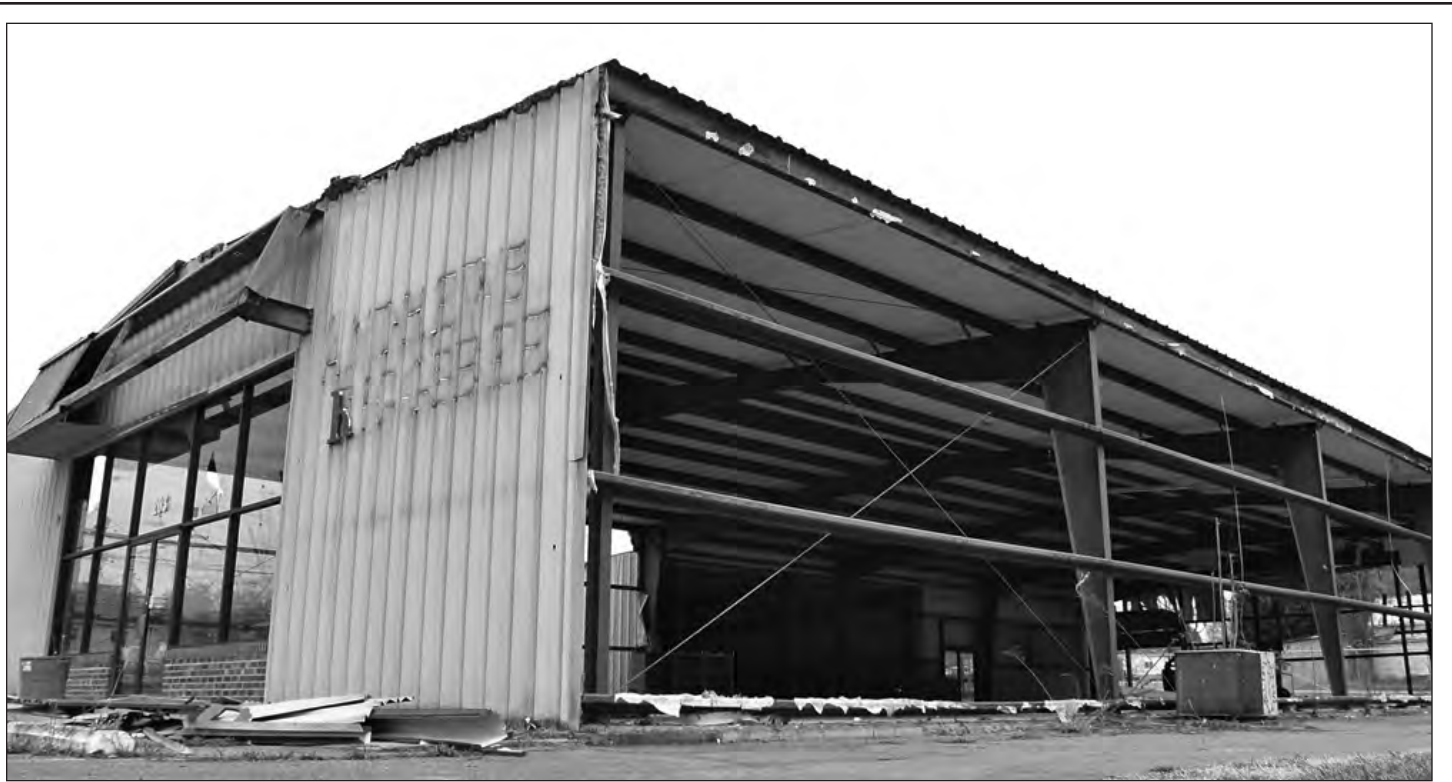
END OF AN ERA — The steel building that was home to Andrews-Riggsbee Hardware started coming down last week to clear the way for a proposed residential and commercial development on the site. No word yet on whether the development will feature a lawnmower repair shop, but don't hold your breath.
