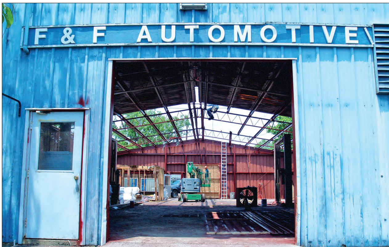
PHOTO BY JORDAN TIMPY The F & F Automotive Inc. building on Weaver Street is undergoing extensive repairs to fix the damage caused by a fire on November 8, 2007. F&F has been a Weaver Street staple since 1972 and hopes to reopen for business by late 2008.
