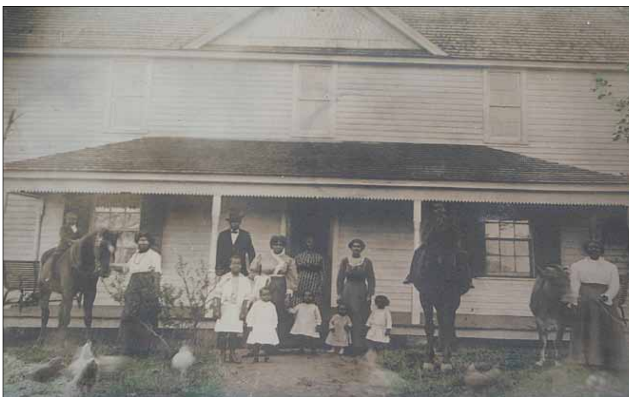
The Strayhorn family in front of their home, which still stands on Jones Ferry Road. This photo depicts the family in the 1930s. Toney Strayhorn was a master bricklayer, and the chimneys and their freestanding corbelled stacks showcase his expertise. PHOTO COURTESY OF DOLORES CLARK
