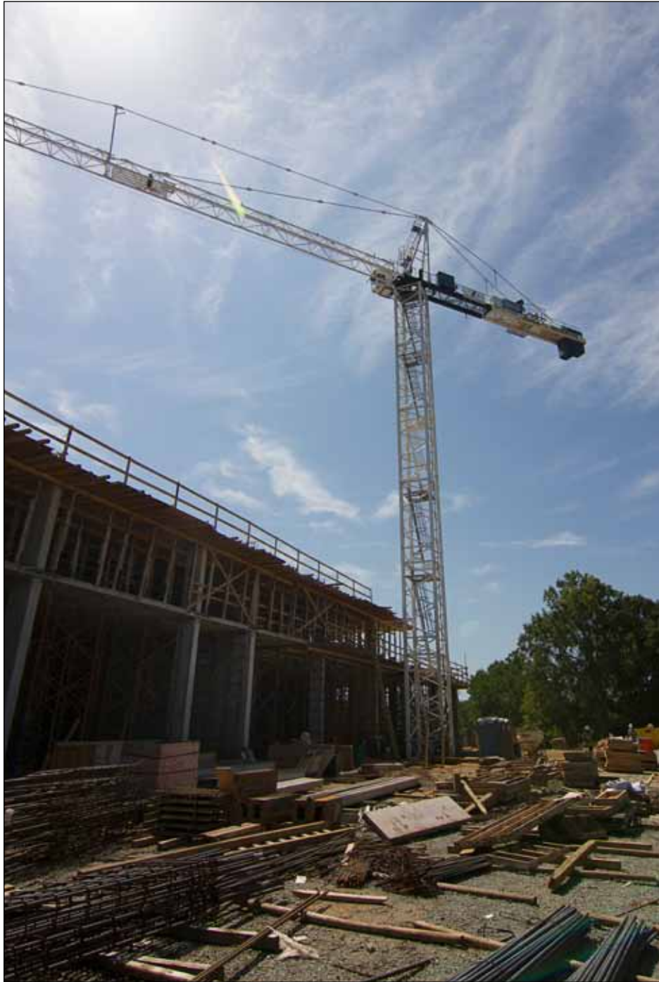
Construction on 300 East Main is progressing on schedule following the March groundbreaking. The crane will likely remain on the site through September.
