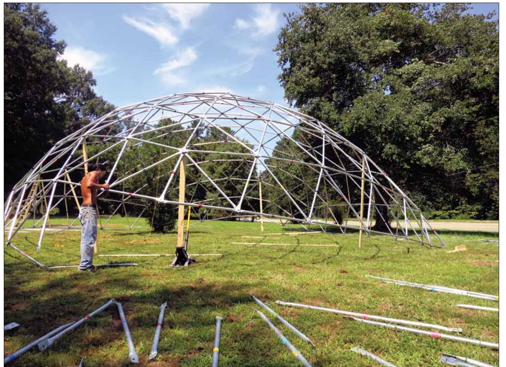
Carrboro resident John Quick deconstructs the geodesic dome he and a few friends constructed to transport out to Nevada's Black Rock Desert for Burning Man, where it will serve as a temporary venue of sorts. PHOTO BY JAMIE DEGRAW
