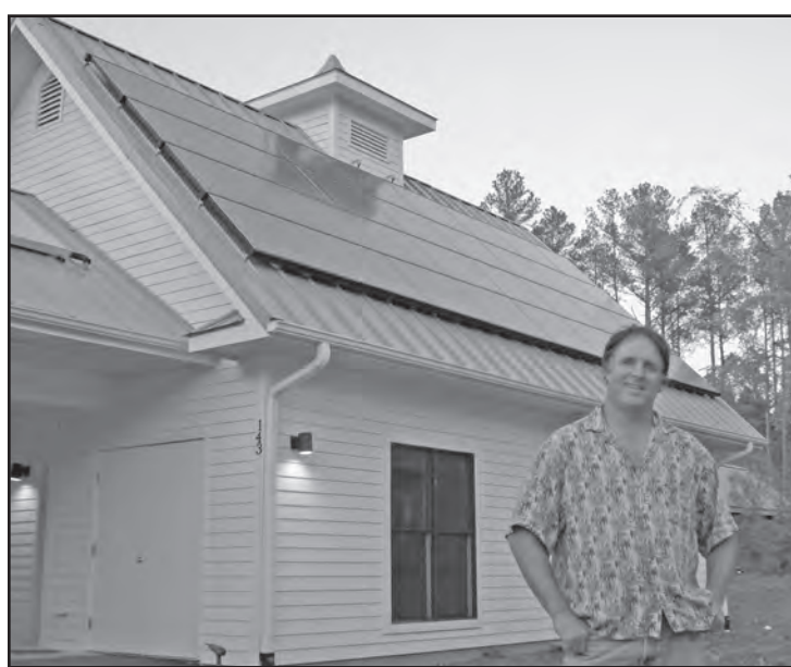
PHOTO BY JACK CARLEY Ed Witkin stands in front of the Pacifica Common House. On the roof, the 5,000 watt solar array he installed converts sunlight to electricity.
