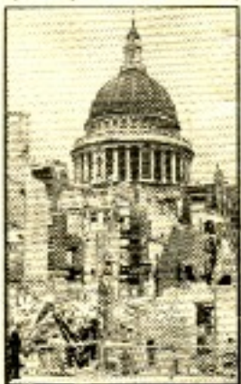
Ministers met here to keep St. Paul's Cathedral looking after the heart of the city. Many Londoners never had such a good view of this famous building, and seldom.
