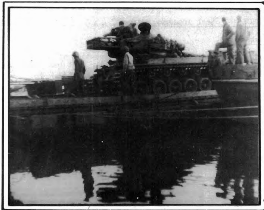
REINFORCED 6 PONTON RAFT
