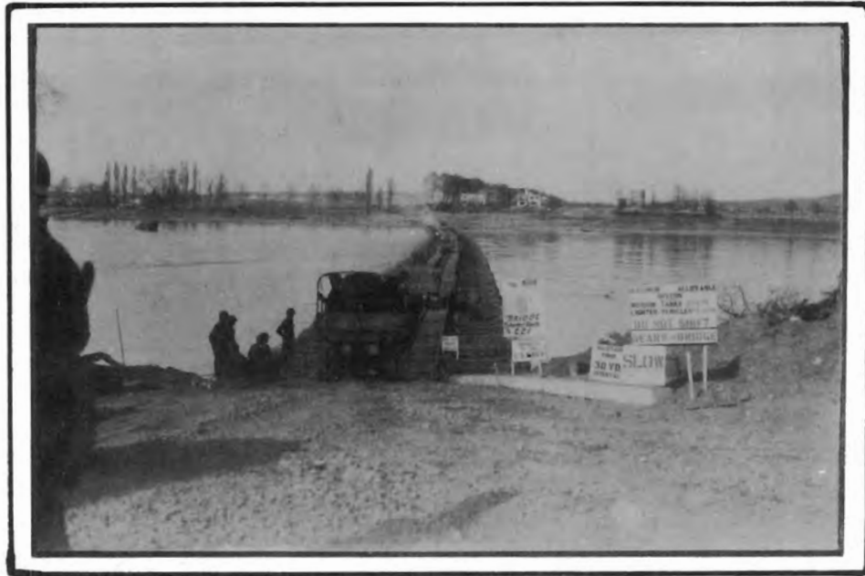
M-2 STEEL TREADWAY BRIDGE
