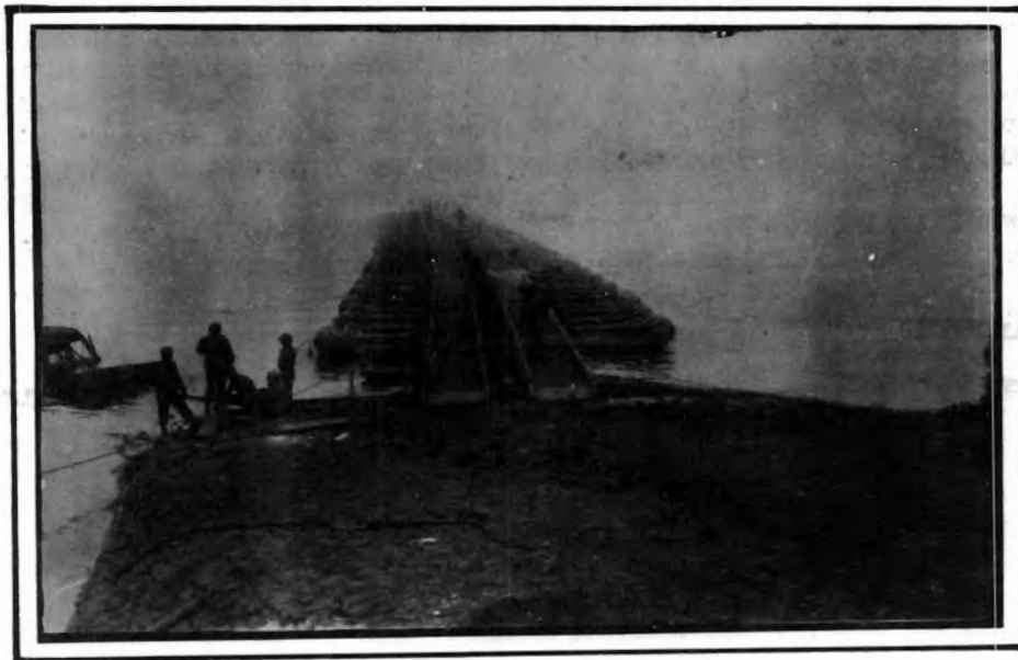
M-2 STEEL TREADWAY BRIDGE
