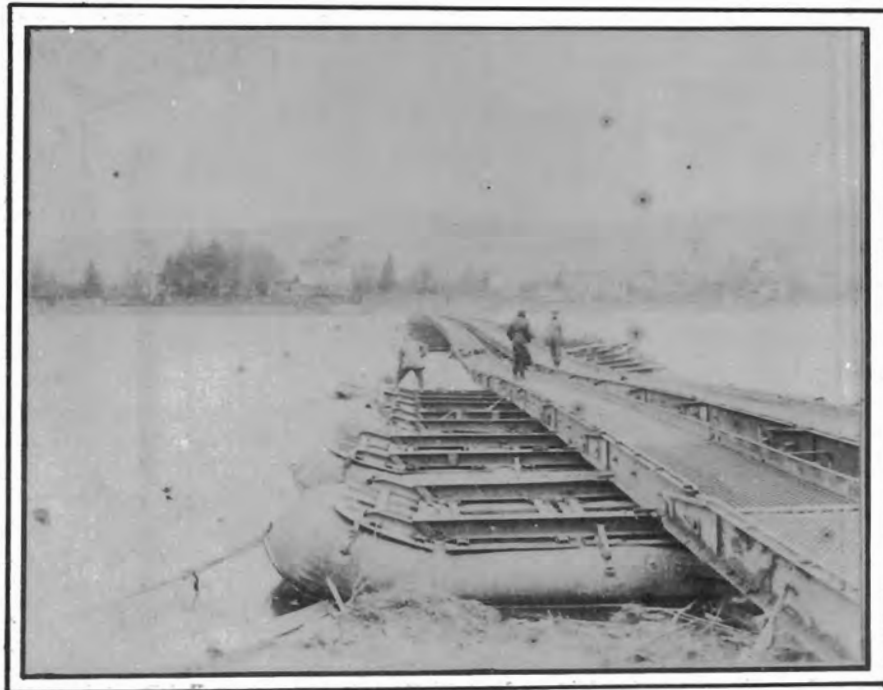
M-2 STEEL TREADWAY BRIDGE
