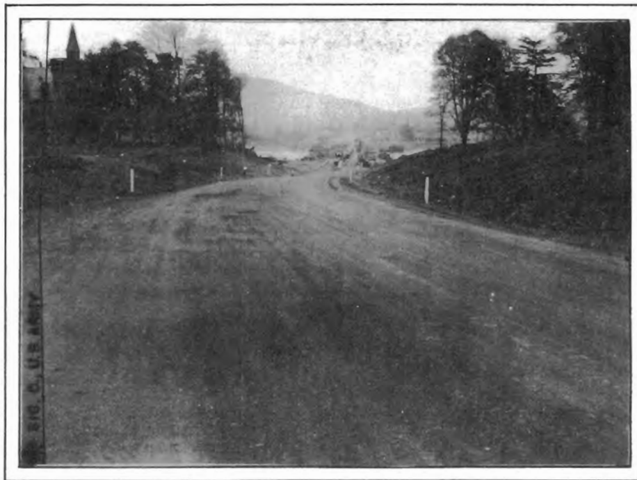
Completed West Shore Approach.
