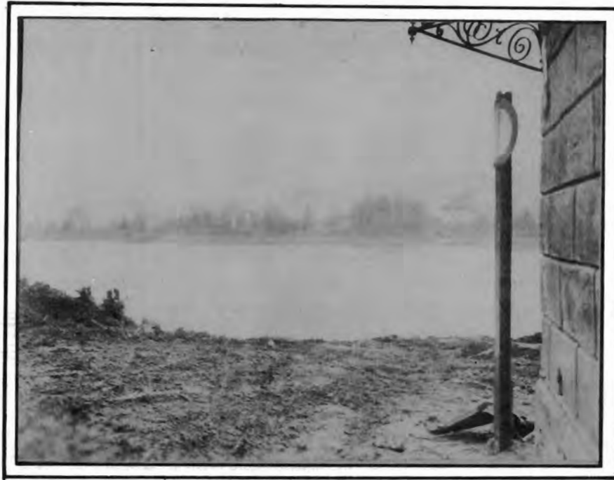
BRIDGE SITE, M-2 TREADWAY BRIDGE
