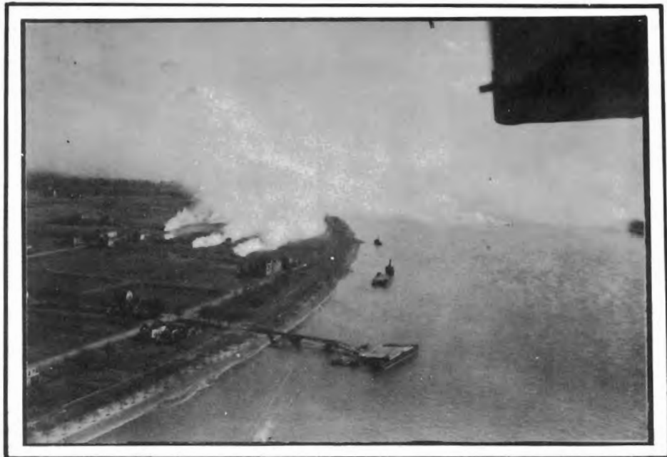
M-2 STEEL TREADWAY BRIDGE
