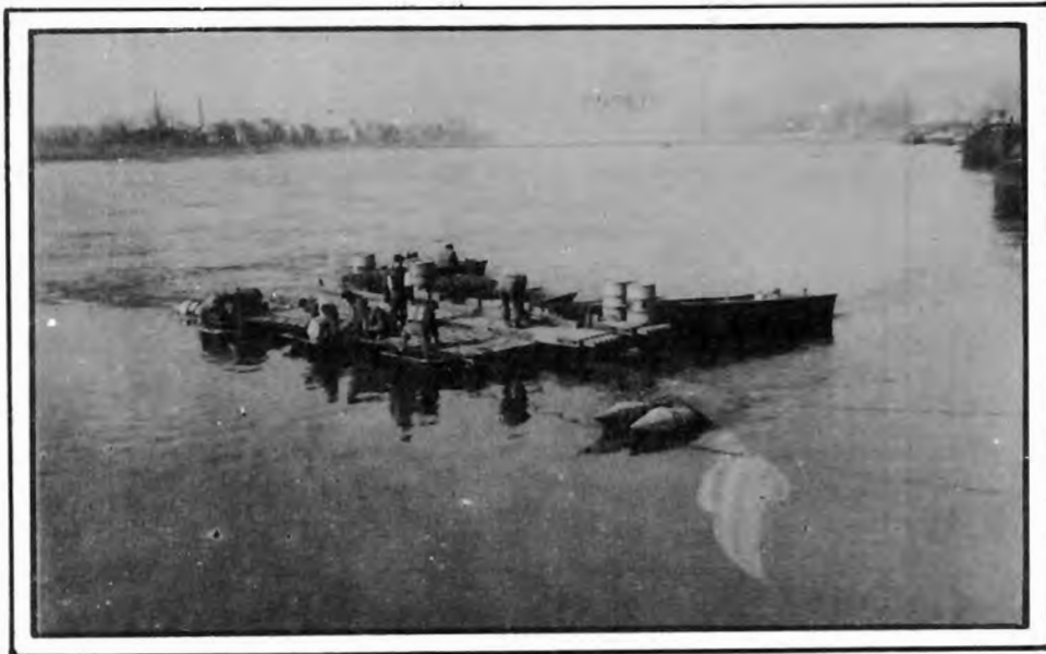
Attaching mine net to jackstays showing use of infantry support raft.
