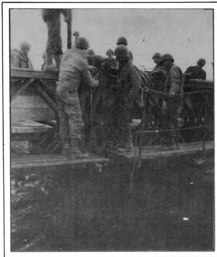
Removing Chain Hoists following connection of Two Bays of Bridge.
