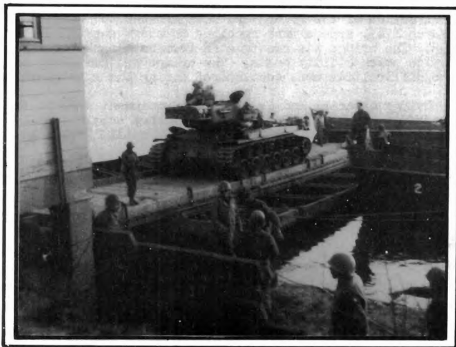
REINFORCED 6 PONTON RAFT
