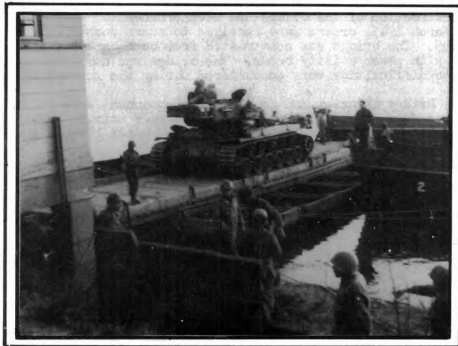
REINFORCED 6 PONTON RAFT
