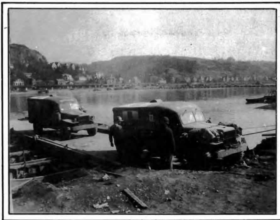
6 PONTON FERRY RAFT
