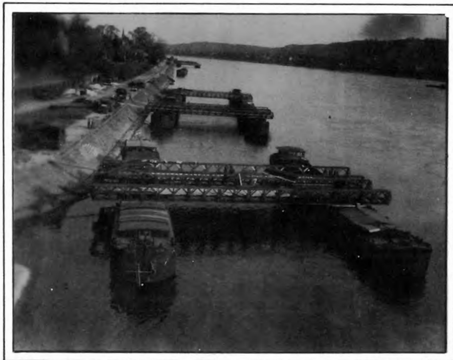
Floating Bays nearing completion.
