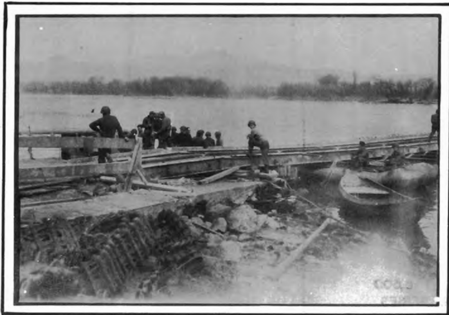
M-2 STEEL TREADWAY BRIDGE
