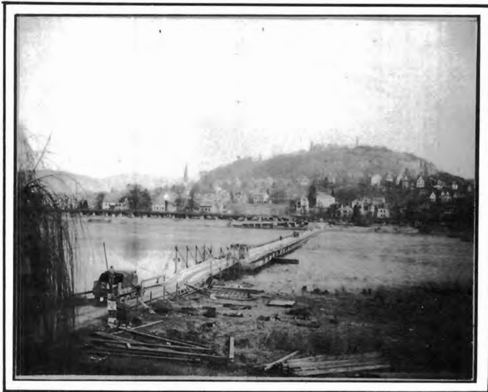
REINFORCED HEAVY PONTON BRIDGE KRIPP, GERMANY, Completed view of bridge from upstream bank of west shore.
