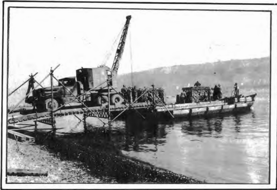
Loading Rubble Box anchors on reinforced heavy ponton rafts. The landing trestles are needed to permit the sea mule to bring the barge into shore without grounding.
