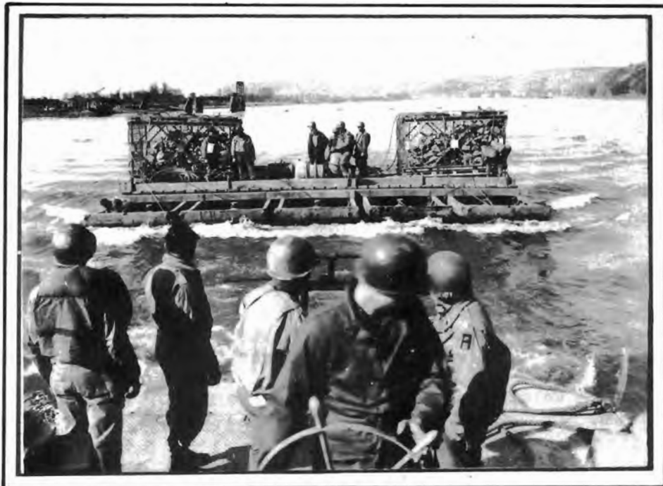
Sea mule towing ponton raft loaded with two Rubble Box anchors. Note high bow wave set up and small amount of free board left.
