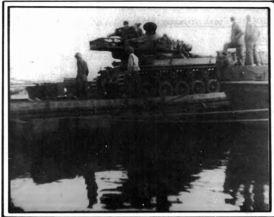
REINFORCED 6 PONTON RAFT
