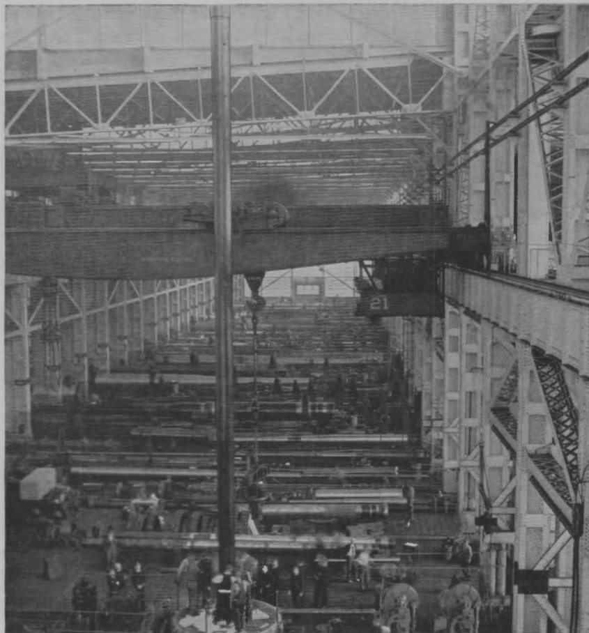
Liner covered with graphite ready to be lowered into hot gun.
