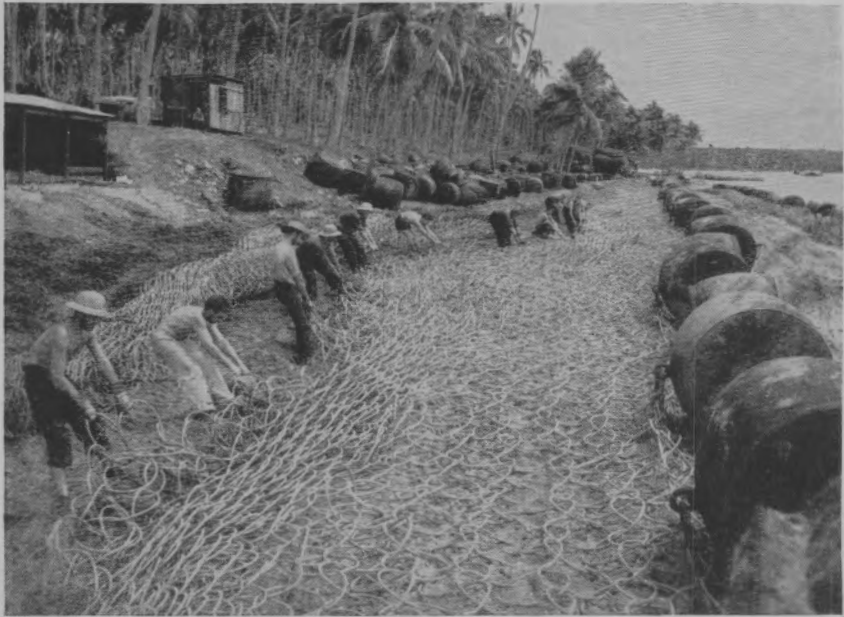
Advanced base detail assembling torpedo net.
