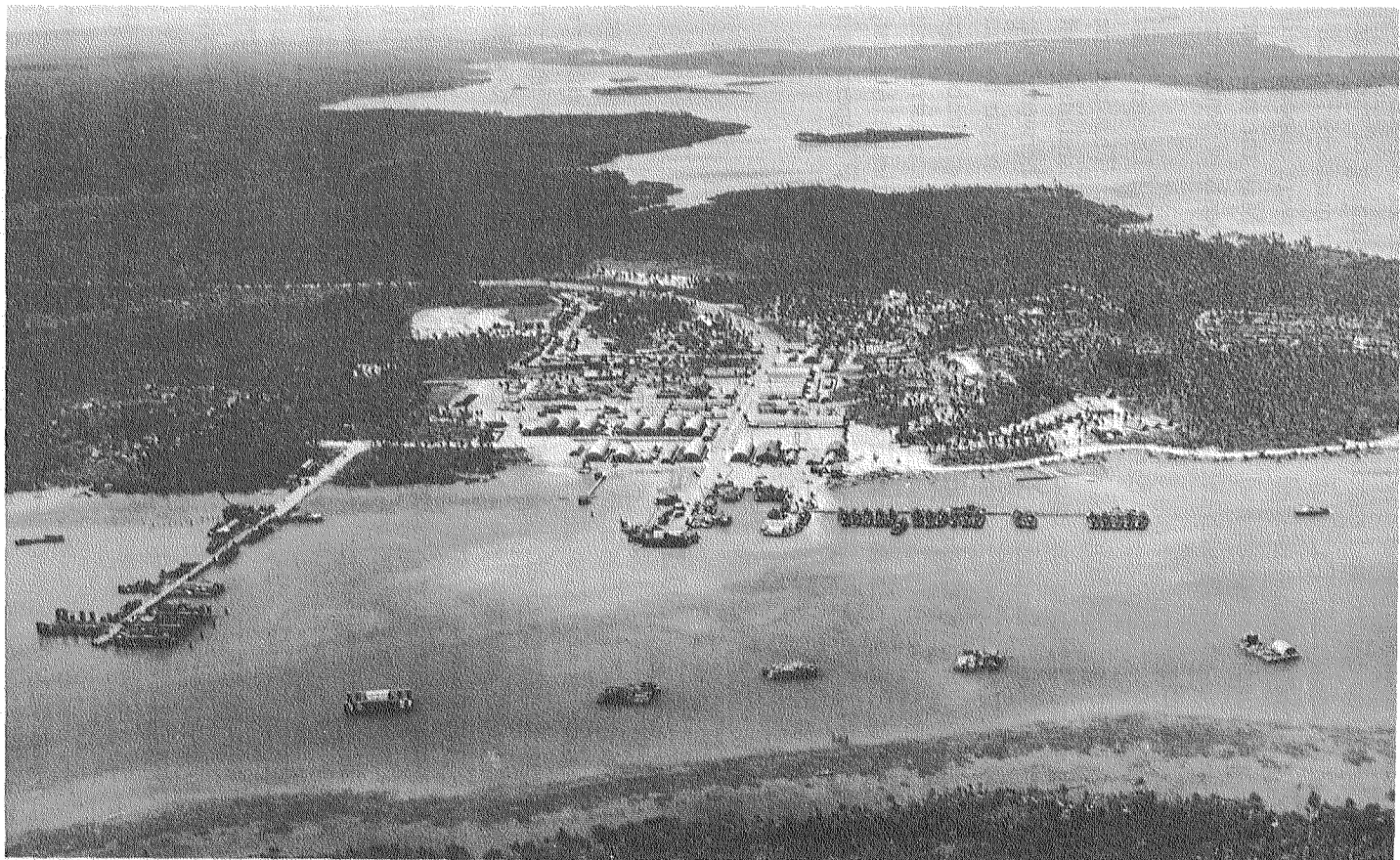
PT Base 17, Bobon Point, Samar.
