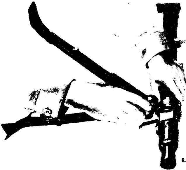
Figure 6 – Mounting Machine Gun on Bipod
