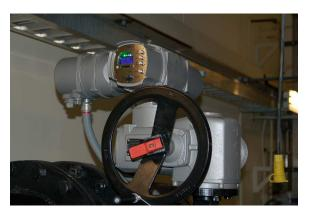
The electronics used within modern MOVs can be quite sophisticated, in some models implementing servo-style control of the motor for precise positioning of the valve mechanism, as well as recording diagnostic data such as motor current which may indicate impending valve mechanism problems like wear and poor seating.
