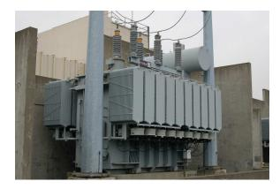
Although transformers have no moving parts, they nevertheless require periodic maintenance and troubleshooting. Maintenance often entails monitoring the chemical composition of their internal oil fill fluid, calibrating temperature sensors and temperature switches, occasionally re-wiring "tap" settings on the windings to compensate for changes in power system loading, etc.
