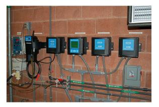
Like all sensing instruments, these require routine calibration to ensure measurement accuracy.
