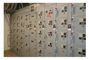
Historically electromechanical in nature, modern MCCs are heavily electronic-based, with electronic motor current monitoring, digitally networked start-stop and speed control for motors, and other features.
