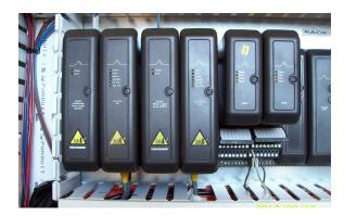
Another photograph shows a much larger-scale DCS, also consisting of electronic modules plugged into a rack:
