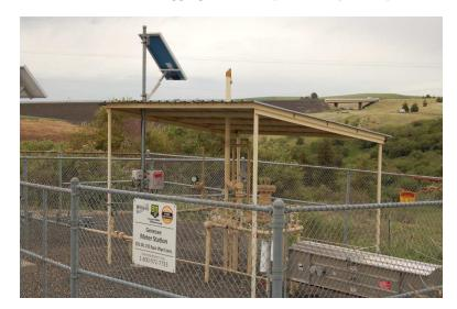
A rechargeable battery provides power to the electronics at night when there is no sunlight, and is recharged by solar energy during the day. This way, the gas pipeline's pressure may be continuously monitored with no ordinary electric power service.
