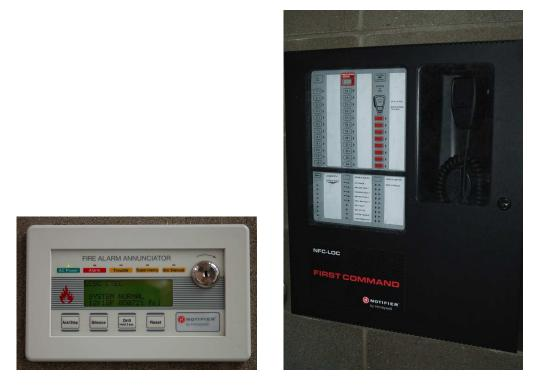
Like HVAC systems, modern fire alarm systems use digital network communications to link multiple devices (e.g. pull-switches, sirens, beacons), each device having its own address number to distinguish it from others on the same network.
