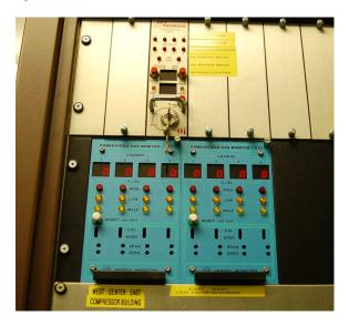
The combustible gas units shown in the above photograph are actually the electronic signalconditioning units for remote-mounted gas sensors, the latter placed close to likely sources of gas leakage or inside of safety-critical areas.
