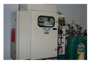
Some gas analyzers exist to detect the presence of hazardous gases in ambient air, such as these combustible gas monitor systems shown below:
