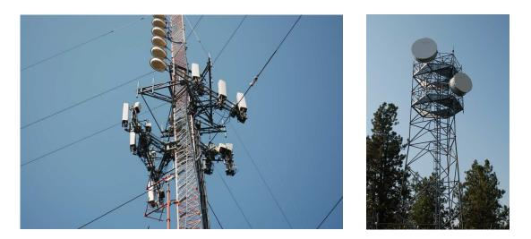
The tower on the left holds cellular telephone antennas (lower) and FM broadcast antennas (upper). The tower on the right holds covered microwave "dish" antennas for high-speed data communication.
