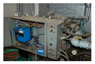
In addition to central control modules such as shown above, there also exist peripheral electronic amplifiers and other units designed to condition signals from flame sensors. An example of a flame sensor amplifier appears below:
