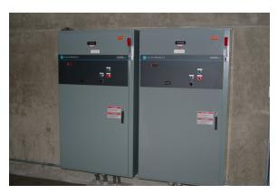
Different types of electric motors require different types of electronic controls to vary their speed. Here we see a photograph of a large motor speed controller for a DC rather than AC electric motor. The industrial application here is driving parts of a paper machine which converts wood pulp into sheets of paper:
