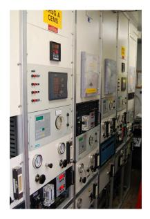
In addition to being complex electronic devices, these gas-analysis instruments are also complex piping and optical systems too. Their maintenance and troubleshooting requires a high level of skill and technical knowledge spanning multiple disciplines.
