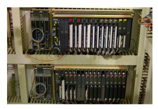
PLCs are especially designed to interface with a great many discrete and/or analog electronic devices such as sensing switches, relays, indicator lamps, analog sensors, etc.
