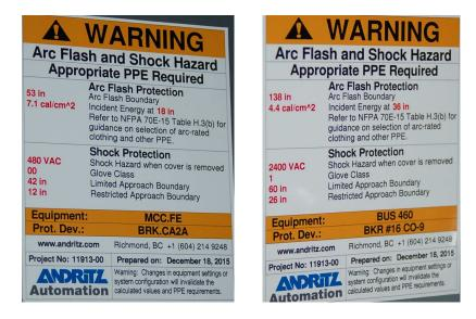
The first line of defense against arc flash is the same as for electric shock: *de-energize the circuit* so there will be no electrical energy present to harm you. The procedure for de-energizing includes placing a warning *tag* as well as a secure *lock* on any main disconnecting switches or circuit breakers to ensure power does not get accidently applied to the circuit while people are in harm's way. This is referred to in industry as *lock-out*, *tag-out*, or *LOTO*.
