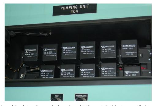
This modular design allows each alarm channel to be serviced without necessarily interrupting the function of the other channels in the annunciator panel.
