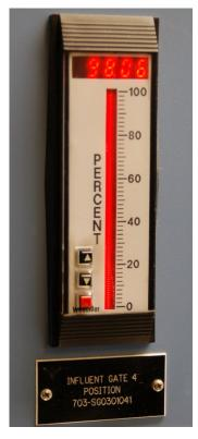
This particular indicator shows the position of a flow-control gate in a wastewater treatment facility, both by numerical value (98.06%) and by the height of a bargraph (very near full open – 100%). It is directly wired in series with the same 4-20 milliamp current signal sent to the gate actuator.
