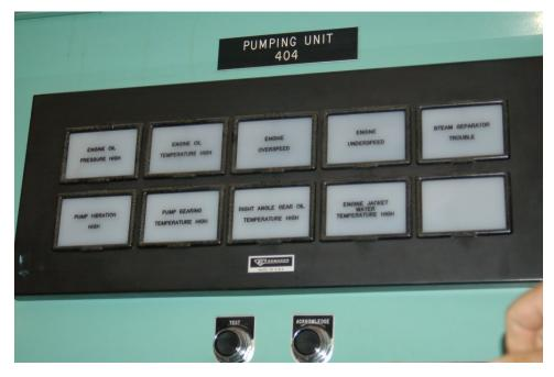
Note the two pushbutton switches below labeled "Test" and "Acknowledge." Pressing the "Acknowledge" button will silence the audible buzzer and also turn any blinking alarm light into a steady (solid) alarm light until the alarm condition clears, at which time the light turns off completely. Pressing the "Test" button turns all alarm lights on, to ensure all light bulbs are still functional.
