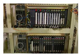
One interesting design feature of most PLCs is the modularity of their I/O. Rather than dedicated pins on an IC serving as input and output channels, PLCs such as this Allen-Bradley PLC-5 support add-on hardware in the form of "cards" that plug into a backplane. These cards may be replaced, upgraded, or swapped with cards having different functionality, all while using the same processor unit to store and run the logic program.
