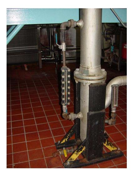
A functional diagram of a sightglass shows how it visually represents the level of liquid inside a vessel such as a storage tank:
