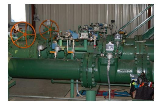
Note the pressure-sensing and temperature-sensing instrumentation installed in the pipe, reporting gas pressure and gas temperature to a flow-calculating computer (along with turbine pulse frequency) for the calculation of natural gas flow rate. Less-critical applications may use a "compensated" turbine flowmeter that mechanically performs the same pressure- and temperature-compensation functions on turbine speed to achieve true gas flow measurement, as shown in the following photograph:
