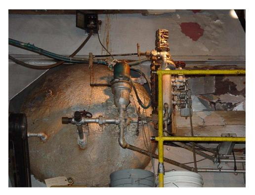
The switch mechanism is a mercury tilt bulb, tilted by a magnet's attraction to a steel rod lifted into position by a float. The float directly senses liquid level, which positions the steel rod either closer to or further away from the magnet. If the rod comes close enough to the magnet, the mercury bottle will tilt and change the switch's electrical status.
