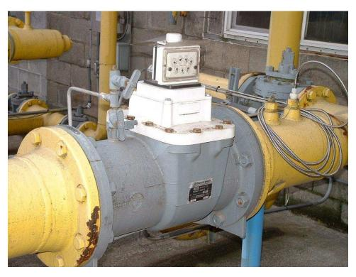
The particular flowmeter shown in the above photograph uses a filled-bulb temperature sensor (note the coiled, armored capillary tube connecting the flowmeter to the bulb) and shows total gas flow by a series of pointers, rather than gas flow *rate*.
