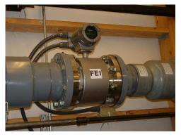
Other magnetic flowmeters have separate electronics and flowtube assemblies, connected together by shielded cable. In these installations, the electronics assembly is referred to as the flow transmitter (FT) and the flowtube as the flow element (FE):
