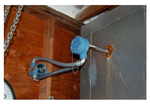
As useful as thermowells are, they are not without their caveats. First and foremost is the firstorder time lag they add to the temperature measurement system by virtue of their mass and specific heat value. It should be intuitively obvious that one or more pounds of metal will not heat up and cool down as fast as a few ounces' worth of RTD or thermocouple, and therefore that the presence of a thermowell will decrease the response time of any temperature-sensing element.
