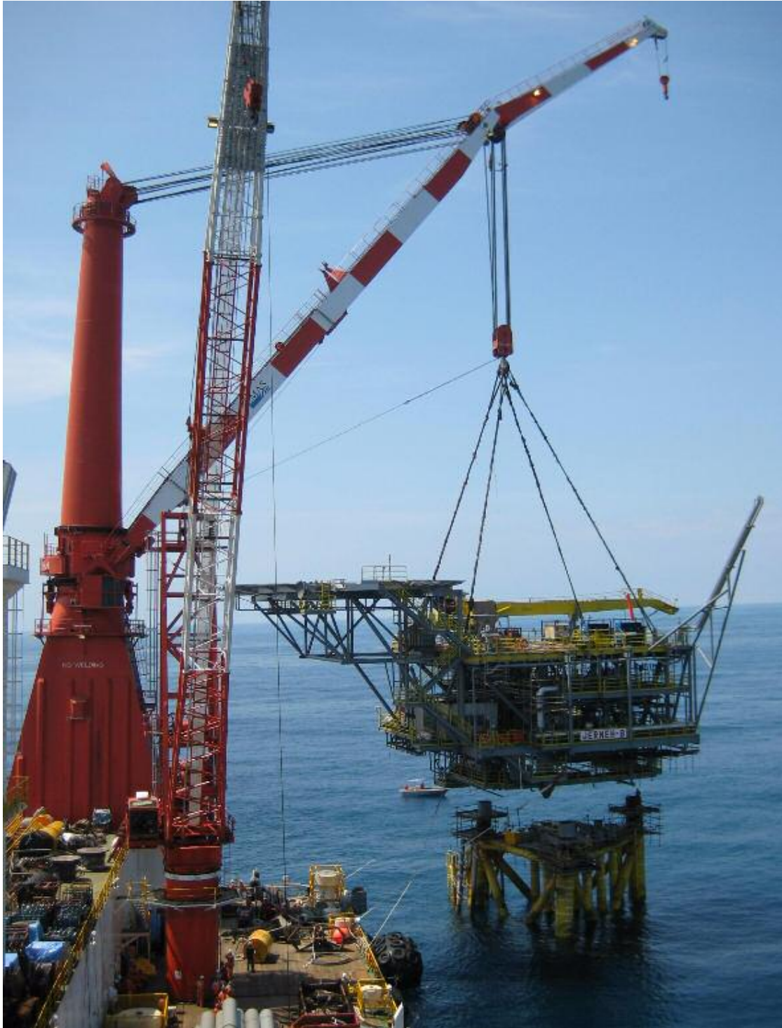
The LEWEK CHAMPION installed the JERNEH-B Topside in the Gulf van Thailand Photo : Flip Geerling - EMAS ©
