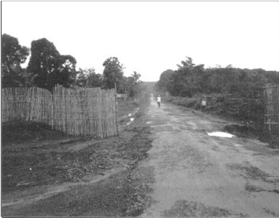
The villages in Southern part of Ye Township are ordered to fence their villages
