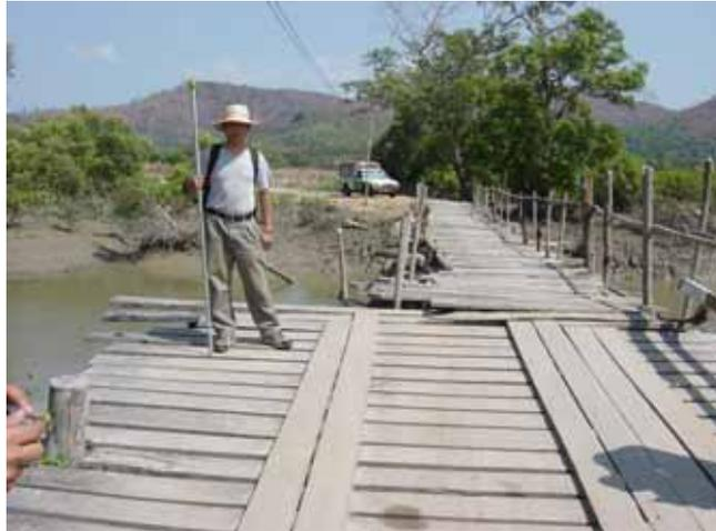
Photo 13 Destruction of bridge to Konnamaing Chaungwa Village by tsunami (narrow flat portion in the right far site of photo)
