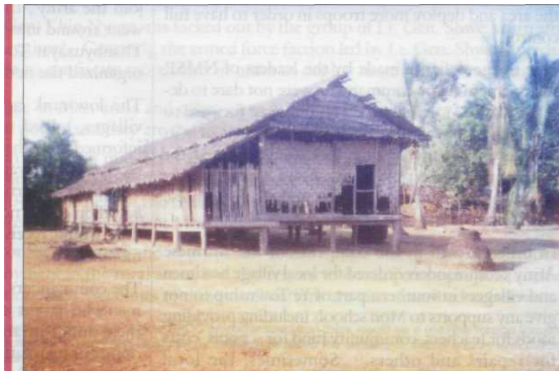
A Mon middle school which is not permitted to repair by SPDC Tactical Commander in southern part of Ye Township.
