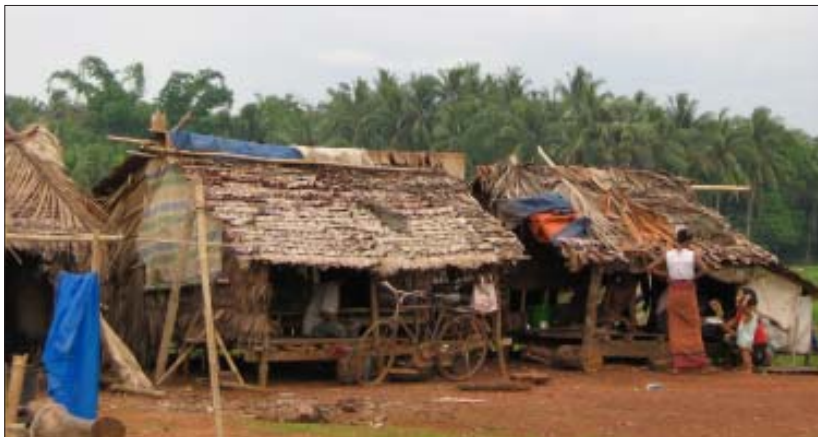
New huts built by the brick makers near Toung-Pyin village, La-mine Sub-Town
