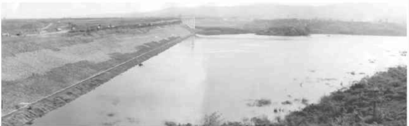
Ma Mya Dam is being built by damming Ma Mya Creek near Hmyinwataung Village in Myanaung Township, Ayeyawady Division.
