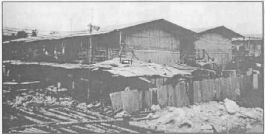
Construction quarters surrounded by unhealthy environment where most construction workers stay
