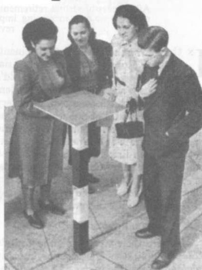
In many streets gas-detectors such as this have been erected. They are coated with a substance that changes colour when gas is about, and then returns to the normal.
