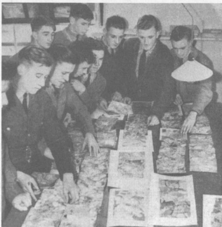
As soon as the reconnaissance aircraft have landed, the exposed films are taken by messenger to a mobile darkroom (above left), and there developed and printed. The map-like pictures are afterwards assembled in a big mosaic, such as the boy apprentices are assembling (above right), which forms a complete plan of the area photographed. The map in page 47 shows a line of division between two photos in mosaic.
