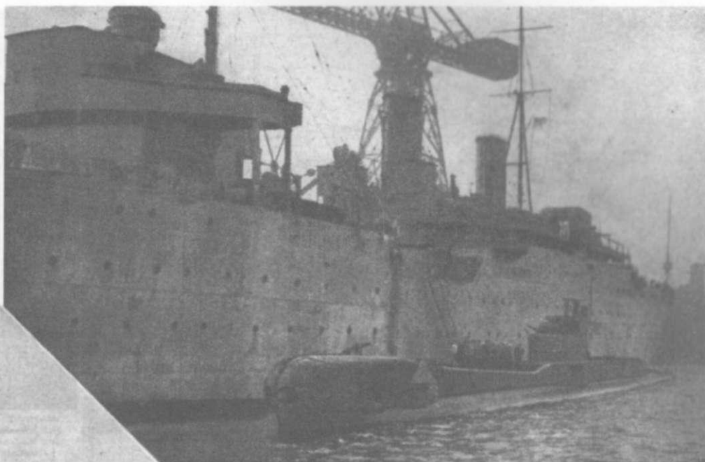
A submarine that has been 17 days on patrol is here coming alongside a depot ship. The largest depot ship in commission at the outbreak of war had a displacement of 14,450 tons, and was designed to "mother" 18 submarines. The man left wears a beard to avoid the difficulties of shaving in his undersea ship.
