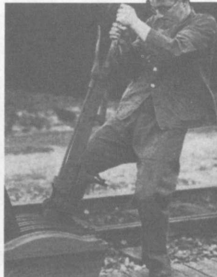
Working the points is an important part of the R.E. railwaymen's training. If pointsmen are not on duty the engine crew may find it necessary to do this work themselves.
