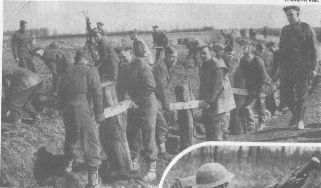
A happy crowd of the Berkshire Regiment now in France apparently find road-making a pleasant change in the "standstill" war. To lay the foundation of a cobblestone road, new work to them, they have devised primitive, but efficient, rammers.
