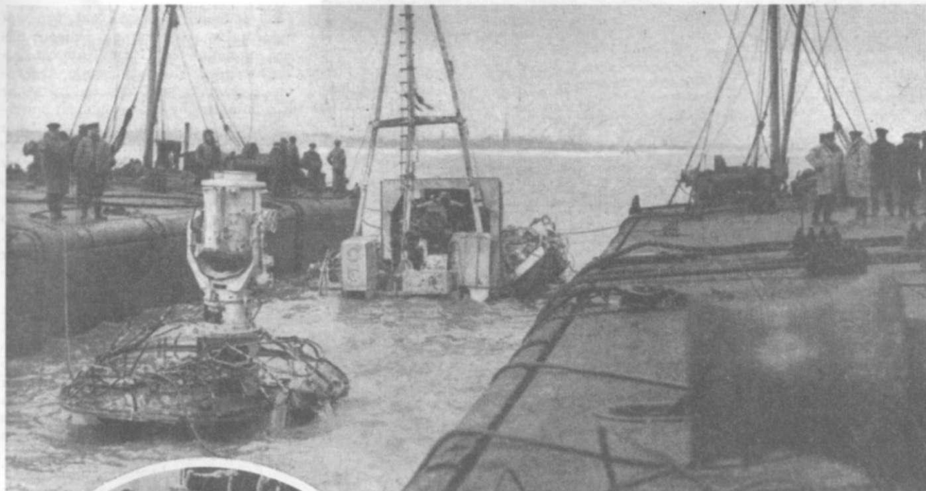
When, on November 21, 1939, the destroyer "Gipsy" struck a magnetic mine off the East Coast it was possible to beach her in shallow water. Later, when the weather was suitable, salvage floats came alongside, as seen above, and she was gradually lifted, tide by tide, until she was in such shallow water that temporary repairs could be effected.
