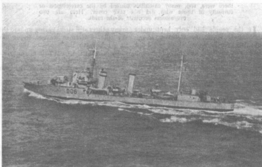
H.M. Destroyer "Keith," sunk by German bombers on June 1, 1940, during the evacuation of the British Expeditionary Force from Dunkirk. The personal narrative of a survivor is given in this page. "Keith" was an Admiralty Type flotilla leader, completed in 1931; her displacement was 1,400 tons, and her speed 35 knots.
