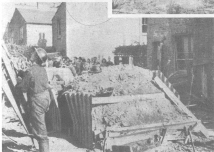
The photograph above shows the necessity of the covering of earth over an Anderson shelter. It was riddled with splinters from a bomb bursting 20 feet away. Left, is a shelter with no earth over the back, a bomb burst 15 feet away and splinters killed two of the occupants.
