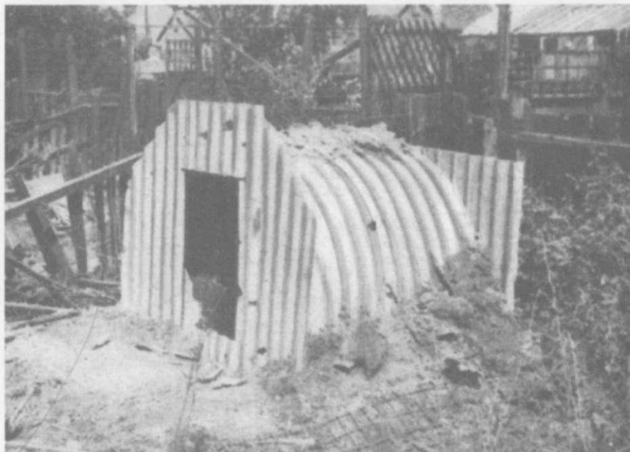
The photograph above shows the necessity of the covering of earth over an Anderson shelter. It was riddled with splinters from a bomb bursting 20 feet away. Left, is a shelter with no earth over the back, a bomb burst 15 feet away and splinters killed two of the occupants.
