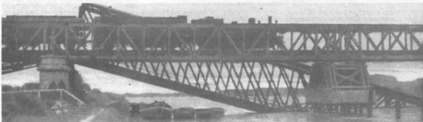
When war clouds first appeared on the horizon, precautions were taken by the French to destroy all the bridges across the Rhine on the frontier between France and Germany. Soon after the declaration of war the bridges were blown up, but after the Armistice one of the first works of restoration undertaken was the building of temporary structures to take their place. Above is one of them built by pioneers in 28 days; beyond it are the remains of the old bridge.
