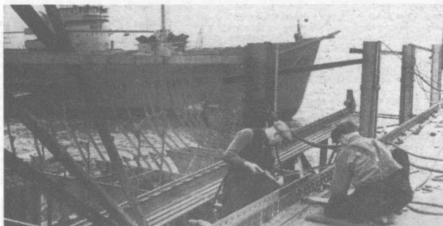
BRITISH SHIPYARDS work at full pressure to make good the losses caused by Hitler's intensive U-boat campaign against our convoys. Riveters are here seen at work on the deck of a new ship at a British shipyard. Beside it the framework of another vessel is shown, while in the background a third ship has been completed and launched. On December 5 it was announced that the U.S.A. was placing 150 merchant ships at Britain's disposal.
