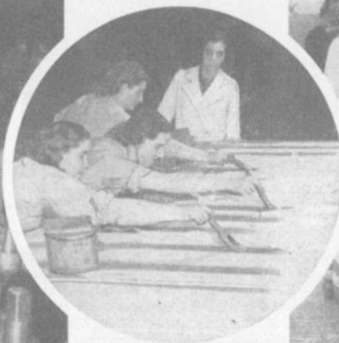
Girl workers (circle) applying dope to a completed wing, the last stage in its construction.
