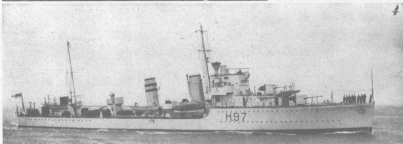
H.M.S. HYPERION, seen in the lower photograph, is of the same class as the five destroyers that took part in the gallant action fought in Narvik on April 11, 1940. She and her seven sister ships were all completed in 1936. They have a displacement of 1,340 tons and a main armament of four 4.7-in. guns and eight 21-in. torpedo tubes. Their speed is 36 knots and their normal complement 145. In the top photograph two destroyers, while at full speed, are making sharp turns to avoid bombs dropped by enemy aircraft.
