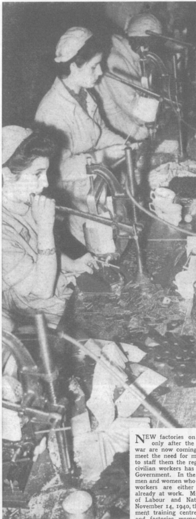
Small parts for bombers are here being made by girls. A jig with holes in the position of those to be bored is clamped over the metal plate. By pulling a lever the drill, revolved by compressed air, is brought in contact. Photo, Fox
