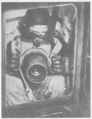
AERIAL RECONNAISSANCE CAMERAS are of two types. One for taking vertical photographs is worked electrically from a fixed position in the floor of the aircraft: one for oblique photographs, as shown above, is manually operated. For an example of a vertical air photograph see Vol. 3, page 590, and for an oblique view, Vol. 4, page 127.
