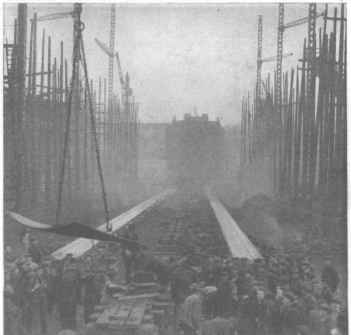
NON-STOP SHIPBUILDING is the order of the day at all British shipbuilding yards. A remarkable illustration of the push being made is afforded by this photograph. A big tanker has just taken the water from the slipway. Before she was towed away to dock for fitting out the workmen, who had paused for a moment to give her a cheer, were again busy getting the keel plate of the next ship into position.
