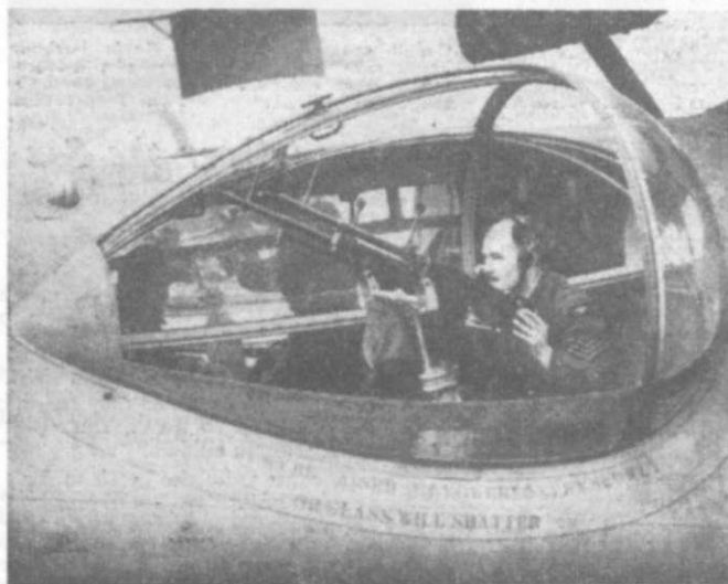
The American-built Consolidated Catalina Patrol Bomber Flying-boat, now in service with the Coastal Command, is fitted with rear gun "blisters," which, as can be seen, give the air gunner a good traverse.
