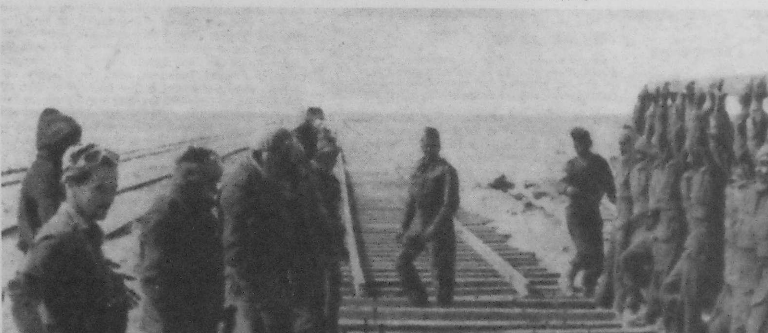
IN LIBYA feverish efforts are being made to speed up communications and augment the existing facilities. New Zealanders are beating all records in laying miles of track across the desert. Below, rails being placed on sleepers for a new track, tanks being taken to the base for refitting on one of the new desert railways.
