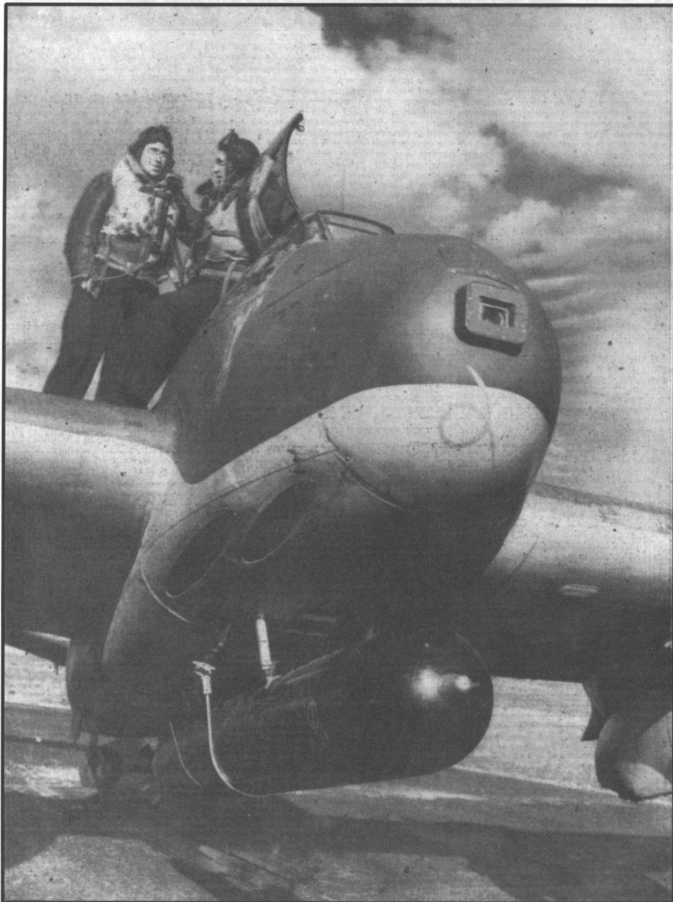
TORPEDO-CARRYING BEAUFIGHTERS , it was disclosed early this year, have been operating with Coastal Command, and have scored great success in attacks against enemy shipping. Armed with four cannon and carrying their "tin fish" under their fuselage, these planes were originally used in the Mediterranean. Two pilots are here shown with a Beaufighter and its torpedo in position.
