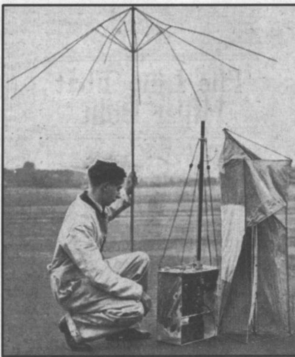
ENEMY SECRETS are sometimes laid bare when aeronautical experts hold post-mortems on captured aircraft. Here is an ingenious apparatus found in a rubber dinghy from a German bomber which had crashed into the sea. It comprises kite, aerial and transmitting set used for sending out S O S signals. Photo, Topical Press
