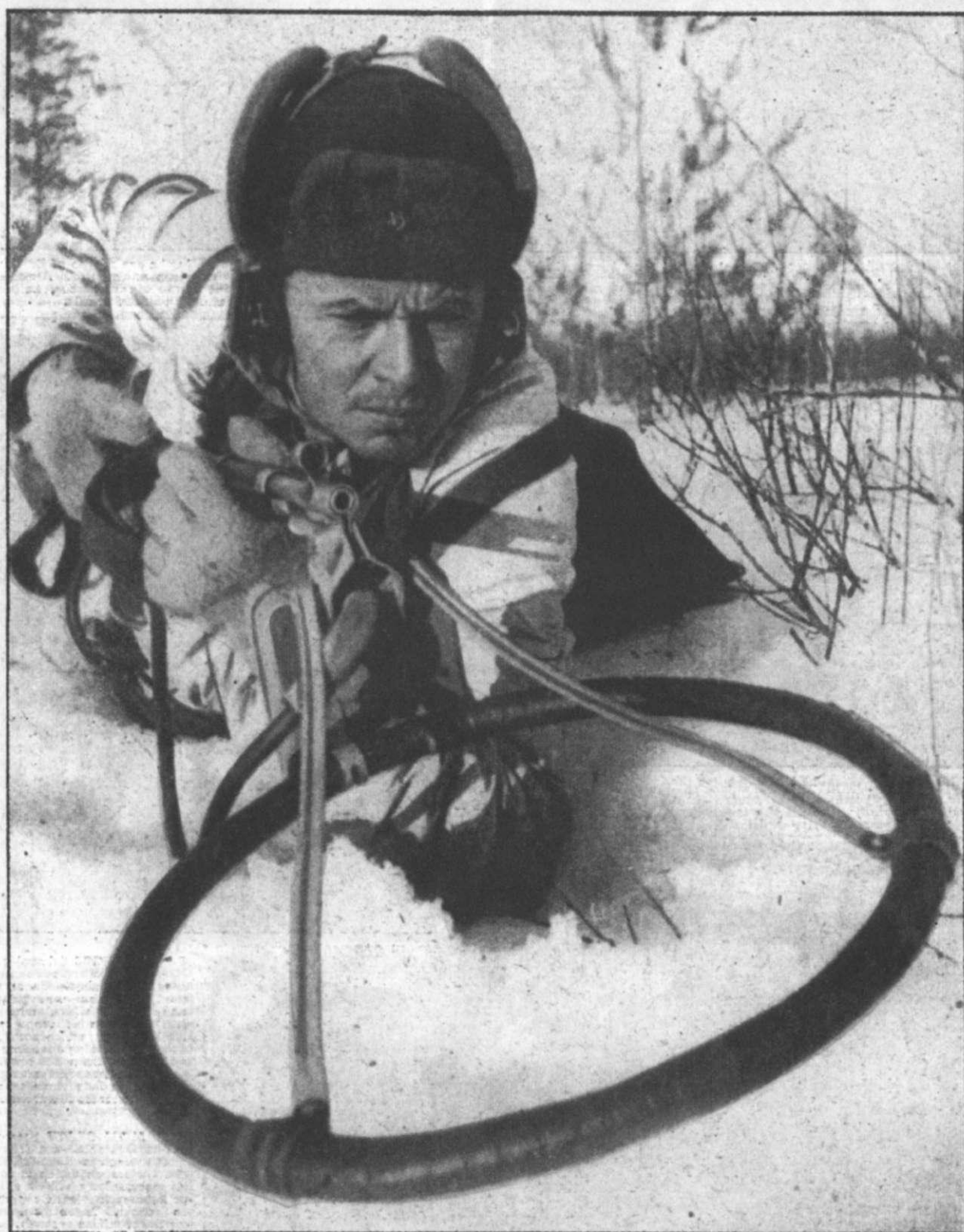
LOCATING ENEMY MINES, this Red Army sapper wriggles along over the snow, pushing his detecting apparatus ahead, seeking shallowly buried explosives left in the wake of retreating Nazis to hinder the Russian advance. Each mine as discovered will be carefully lifted and rendered innocuous. The British method consists in detecting along a "lane" marked through the minefield with tapes; sappers follow, marking each position: then come the men who unearth the mines and remove the detonators. Photo, U.S.S.R. Official
