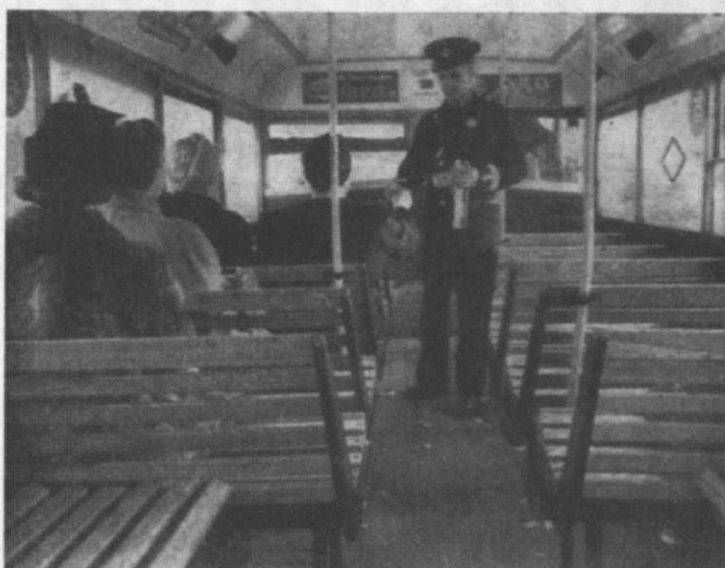
THIS LONDON 'UTILITY' BUS , among the first of its kind, dispenses with pre-war cushioned comfort. Introduced in July 1943, it has wooden slatted seats which have not been seen in London's buses since 1925. There are 65 of these austerity vehicles in use at the present time.
