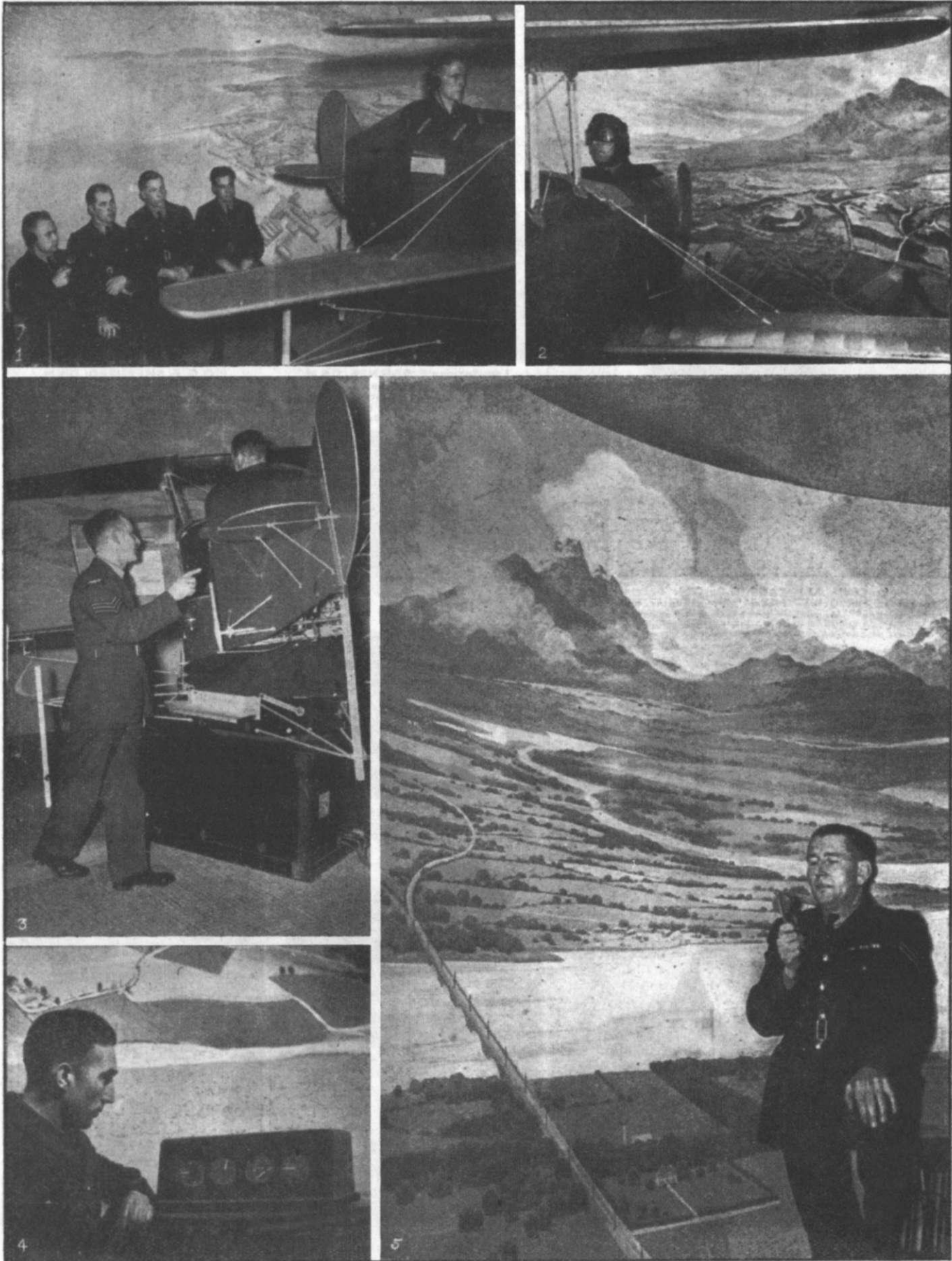
IN THE COCKPIT of a Visual Link Trainer sits a pupil (1) in telephonic contact with an instructor (left), while three other learners watch, near the cyclorama circular screen. Whatever movement the pilot makes he has an aerial landscape before—or rather, through optical illusion, beneath—his dummy plane (2). The instructor explains the Link's controls (3), gives the pupil flying directions by microphone (5), and checks his reactions by meters corresponding with those in the Link (4). See also facing page.
