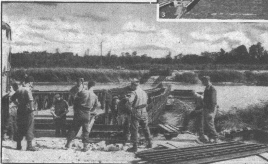
TRIPLE TIER specimen (3) In the first stage in bridging a gap the Bailey is built on rollers on the bank, each span as completed being pushed out and over. Only one steel pin is required for each join.
