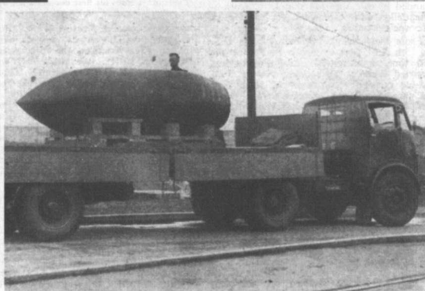
TEN-TON BOMB of the R.A.F. (below) rides to the filling-centre on a specially designed lorry with 90 h.p. Diesel engine. These gigantic missiles softened up the Reich for the big advance. They are flown to their targets in Lancaster bombers, which themselves weigh just over ten tons. See also illus. in page 764.
