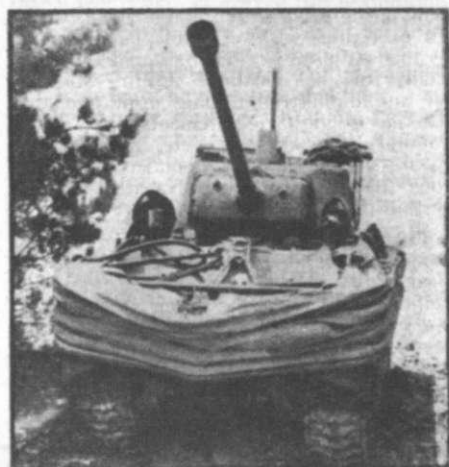
AMERICAN VERSION, after landing, with its canvas "walls" lowered. How this type of amphibious tank assisted in D-Day landings is told here. Photo, Associated Press
