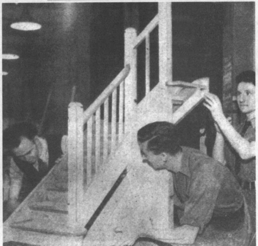
LEARNING TO BUILD TOMORROW'S BRITAIN , ex-Servicemen are training at Eley's Estate, Edmonton, London, where workshops have been erected for them to study various crafts. Much use is made of models: trainees (above) are at work on a model staircase; others (top) are perfecting themselves in bricklaying as appertaining to the construction of railway tunnels and bridges.
