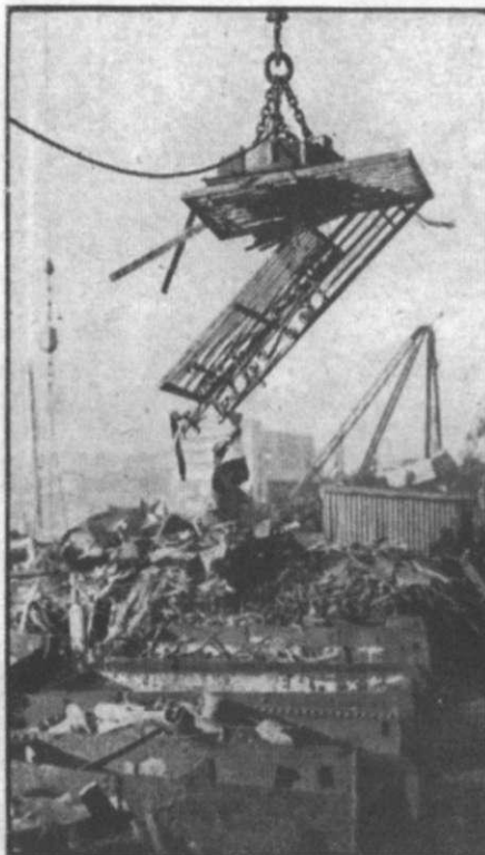
GIGANTIC ELECTRO-MAGNET unloads scrap-iron from a wagon and places it in a bin for later transport to the blast furnaces. During the great salvage drive of 1940, eighty per cent of old iron recovered went to make bombs for the R.A.F. Photo, Topical Press
