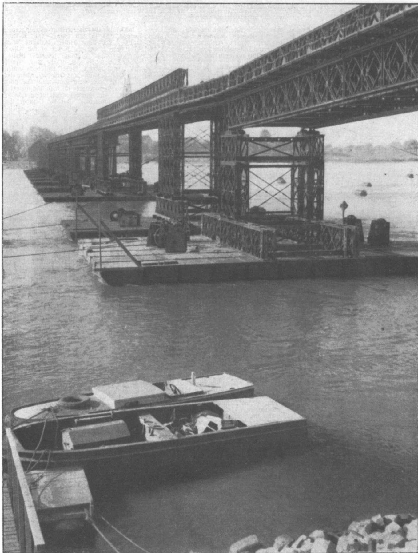
ONE OF THE LARGEST FLOATING BRIDGES IN THE WORLD, across the turbulent Rhine at Düsseldorf, had been almost completed by men of the Royal Engineers in early November 1945. Built as a semi-permanent structure, it is known locally as the "Freeman Bridge," after a major of the R.E.s, who was largely responsible for its erection. This "Bailey on Stilts" is half-a-mile long and can carry loads up to 40 tons. It is the work of three companies of sappers, some of whom learned their craft in Burma. See also pages 564-565, Vol. 8. PAGE 457 Photo, British Official
