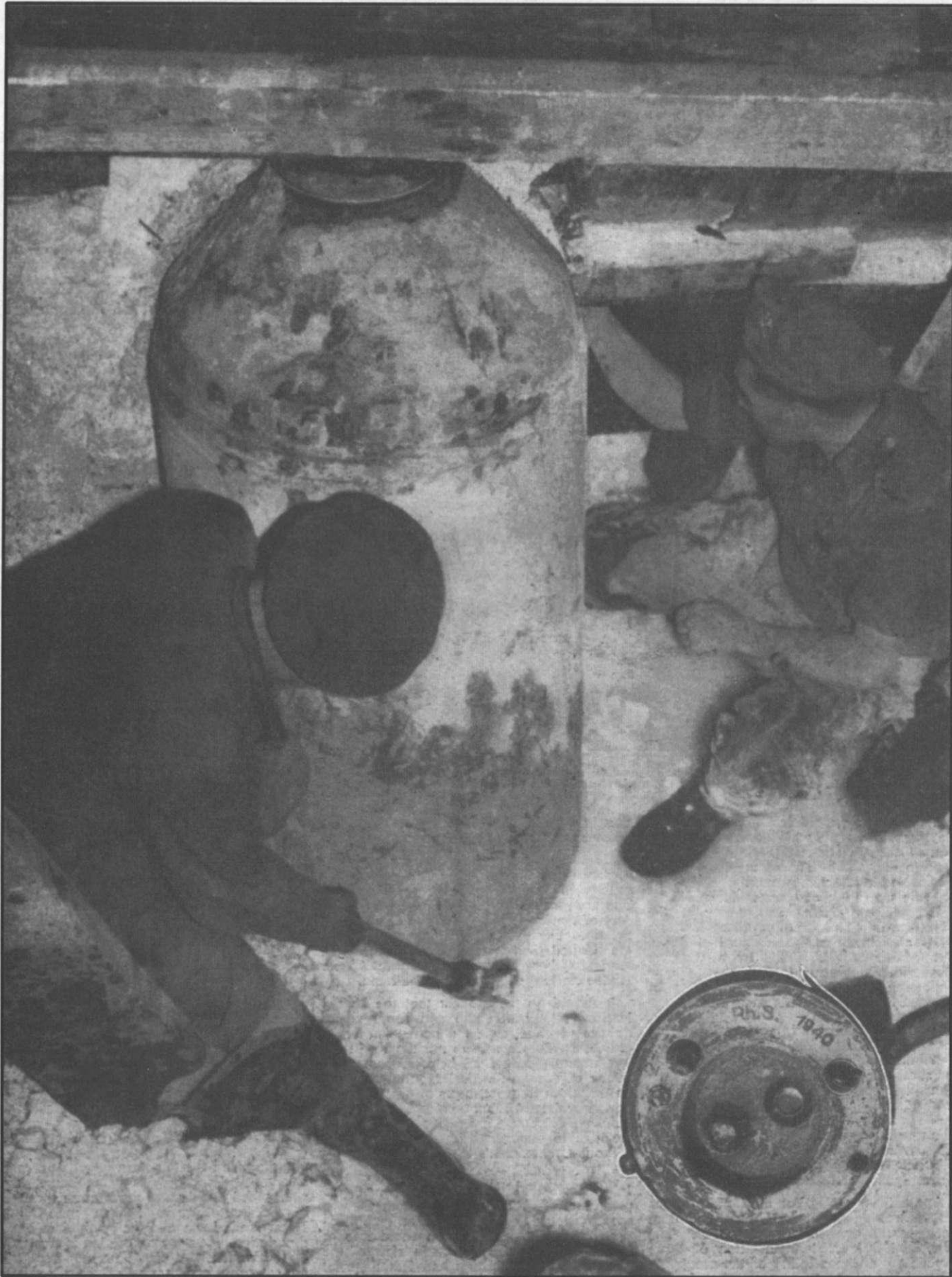
"HERMANN," THE 4,000-lb. LUFTWAFFE BOMB, which buried itself over 40 ft. deep in a Croydon, Surrey, timber yard on January 11, 1941, was finally rendered harmless and removed on December 17, 1945. A bomb disposal squad of 26 sappers of the Royal Engineers completed the task in 200 days, earlier efforts being hampered by an underground stream. During the last stages over a hundred local residents were evacuated. At the bottom of the shaft sunk to find it, two of the sappers are here digging around the bomb. Inset is part of the fuse. PAGE 565 Photos, Associated Press
